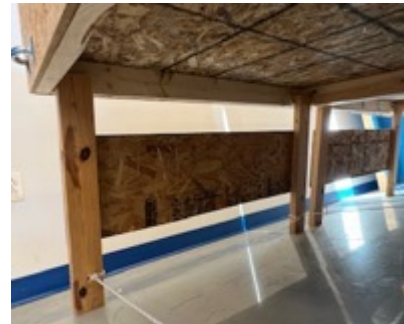
HINGES ALLOW LEG ASSEMBLY TO FOLD FLAT UNDER FLOOR. THE SUBFLOOR FRAME LIMITS THE LEGS FROM EXTENDING TOO FAR.
