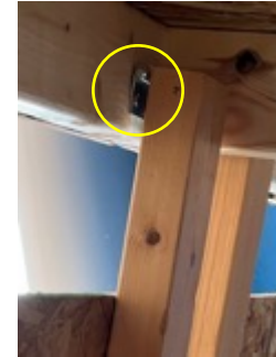
HINGES ALLOW LEG ASSEMBLY TO FOLD FLAT UNDER FLOOR. THE SUBFLOOR FRAME LIMITS THE LEGS FROM EXTENDING TOO FAR.
